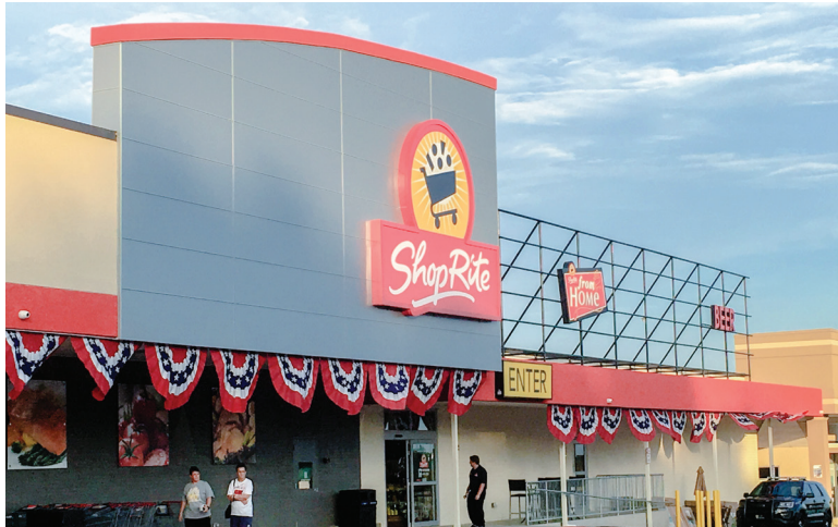
The commercial construction firm has been building grocery stores, like this ShopRite in Brookhaven, Pa., for more than 30 years.
